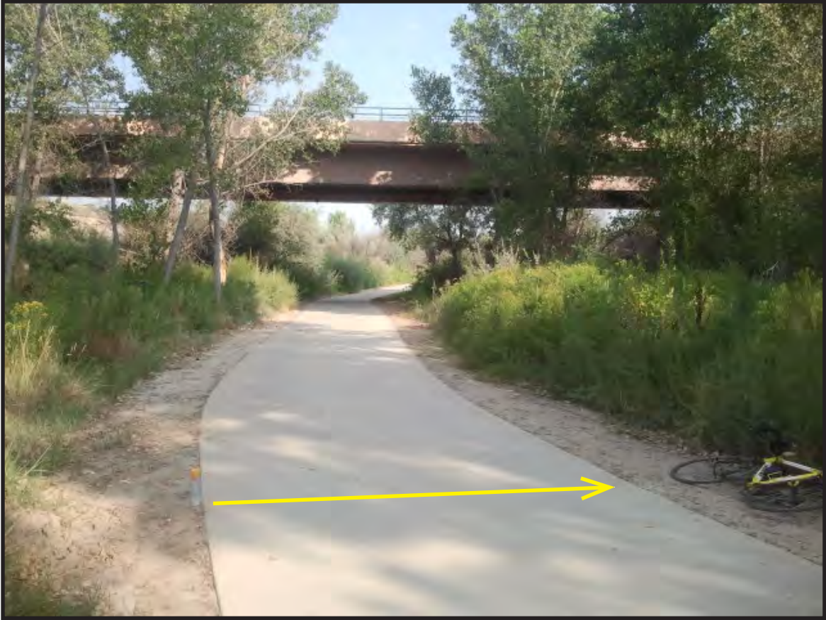
Turnaround, looking northwest
