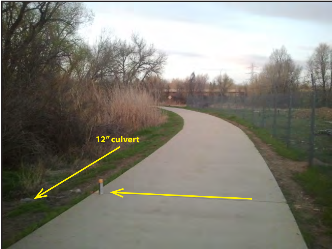
1 mile, looking southwest
